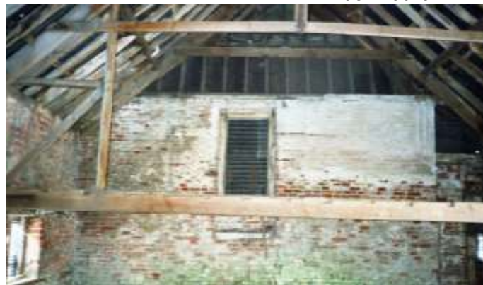
The interior of the kiln and (right) is the kiln from the germination floor - first floor removed and so roof structure visible
