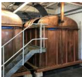
Mash tun and copper wort coolers at the Unicorn Brewery
