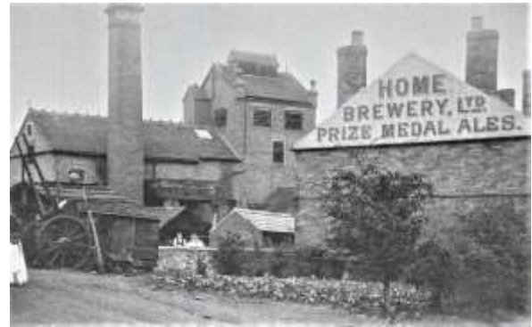
Home Brewery in Evers Street, Quarry Bank. It was originally known as the Swan Brewery, but was taken over by J P Simpkins in 1903 and renamed
