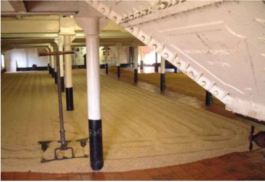
The malting floor at Wolverhampton and Dudley Breweries maltings at Lichfield in 2003
